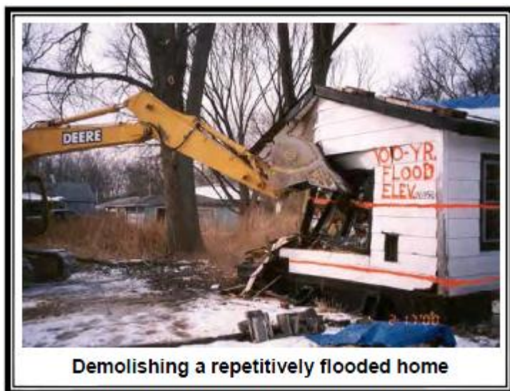
Figure C-5 Demolition of Flooded Home
